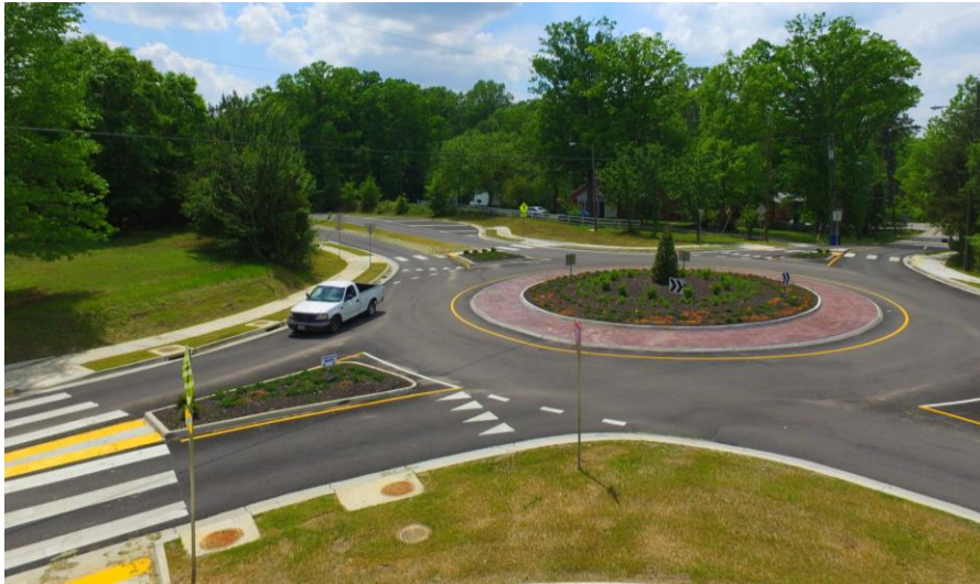
Neighborhood Traffic Circle
